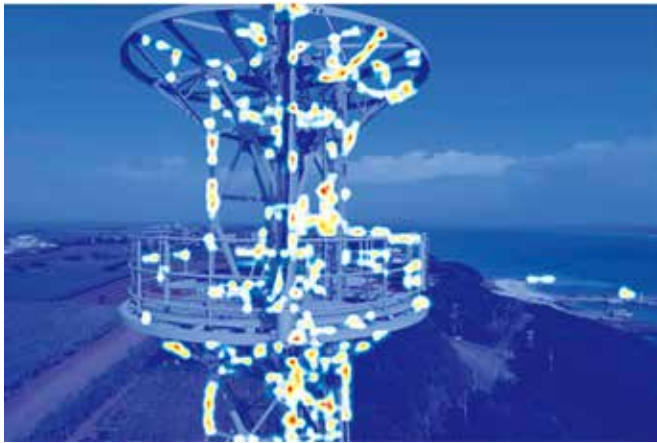
■ Figure 2: Detection of rust
