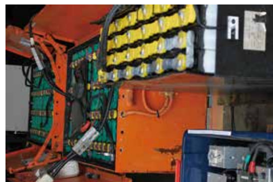
Lead-acid batteries undergoing regeneration charging
