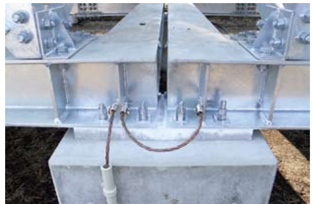
■ Photo 4: Foundations and framework provided with expansion joints
