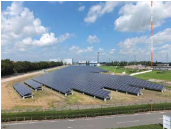
Photo 1: NHK Shobu-Kuki Megasolar power plant
