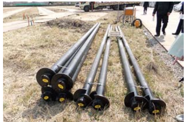
■ Photo 3: Winged steel pipe piles
