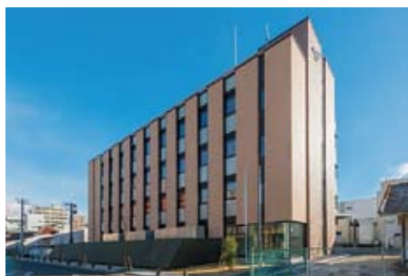
■ Photo 1: The Resilient ICT Research Center
