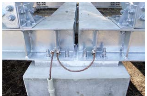
■ Photo 4: Foundations and framework provided with expansion joints
