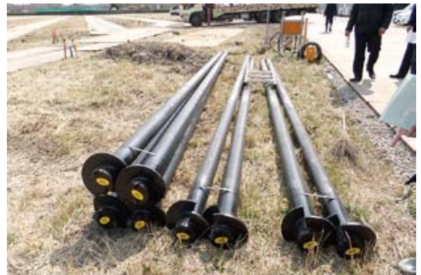
■ Photo 3: Winged steel pipe piles
