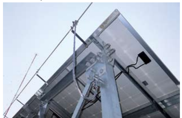
■ Photo 5: Lightning protection system for solar panels
