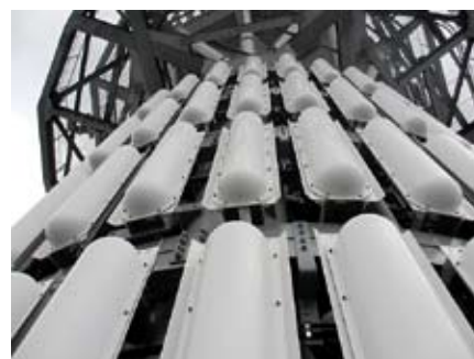
Photo 2: TV transmission antenna
